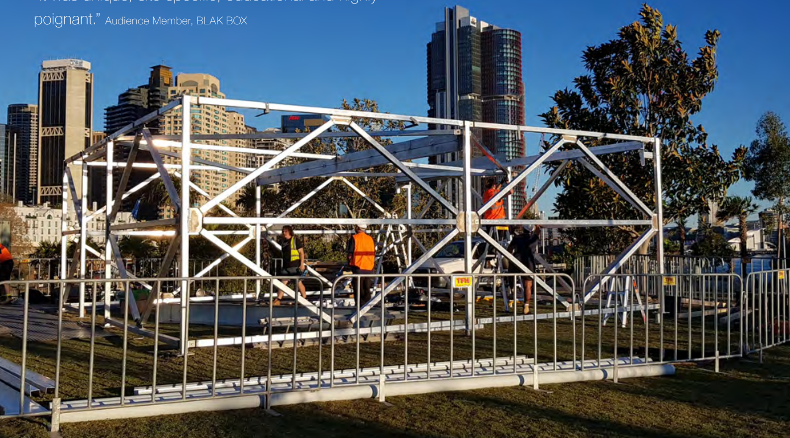
Image Blak Box being installed at Barangaroo. Photographer Kris Spann
